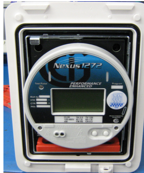
Paddle Board Completely Installed
