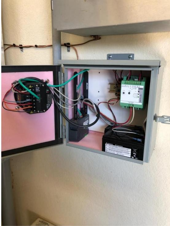
The typical voltage monitoring installation at CPEC consists of a Shark® 200 meter with a V3 switch and a Sierra Wireless RV50 4G cellular router, with UPS to provide meter power and communication capability during outages (See photo on the left).
